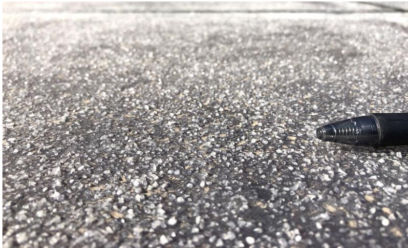
Photo 7 - Leveling the surface of the module.
