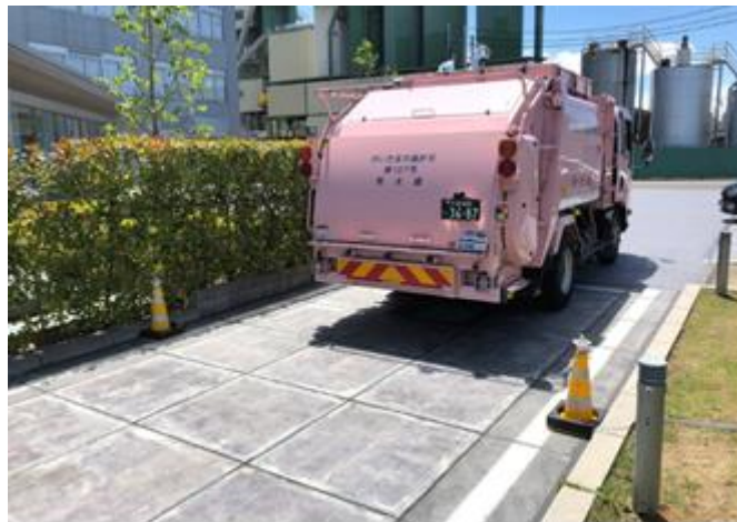
Photo 3 - Laid test pavement.
