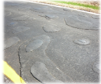
Patched Asphalt Road
