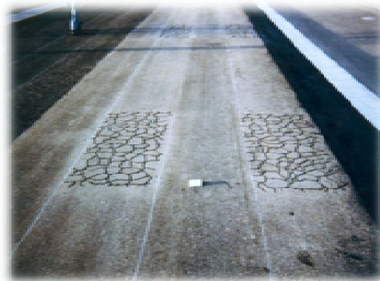
Cracked Asphalt
