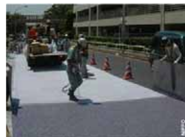
Figure 10 – MMA-type construction
