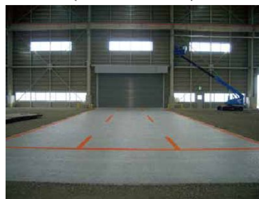
Warehouse Floor (Sendai-shi, Miyagi)
