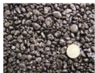
Surface of open graded asphalt concrete base
