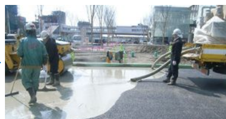
Grouting POLYSEAL GROUT
